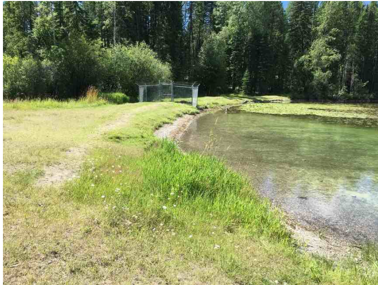
Photo 2.1 Tie Lake Dam – Looking west. West side of dam. Note remnants from 2012 sandbagging.
